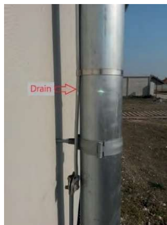
Fig. 3. Drain fixed on a vertical gutter pipe 7)
