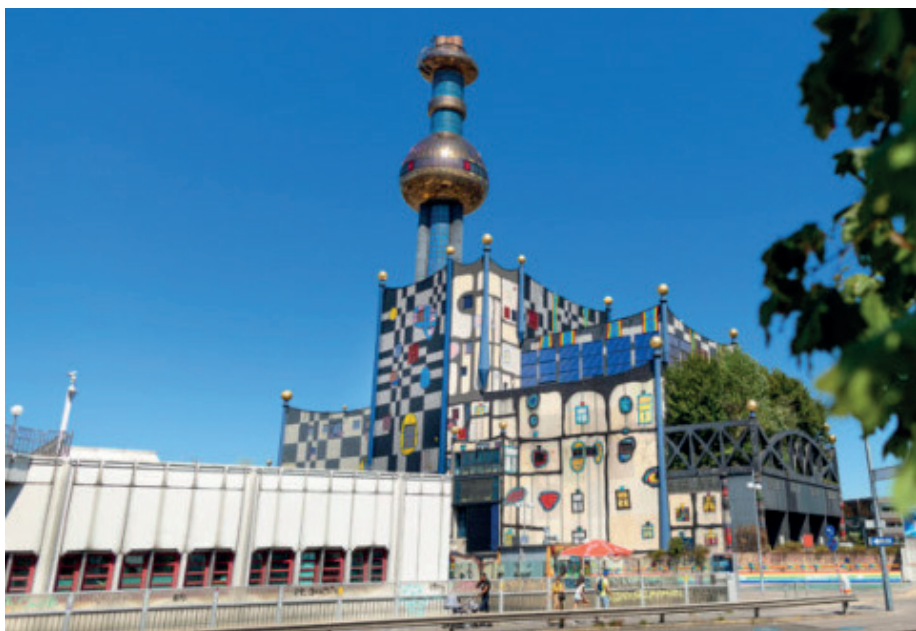
Fig. 8. Waste-fired communal heat and power station in Wien Spittelau 27)
